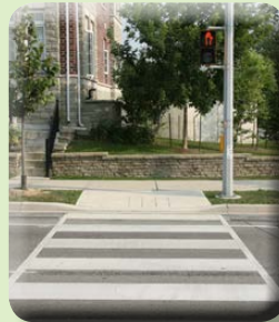
Enhanced Pedestrian Crosswalk Markings
