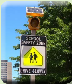
School Safety Zone Signs with Flashing Beacon
