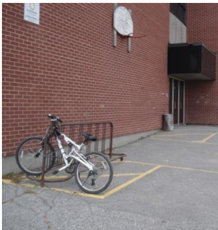
Existing bike rack
